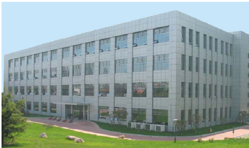
Ligent Photonics Manufacturing Facility Qingdao, China
